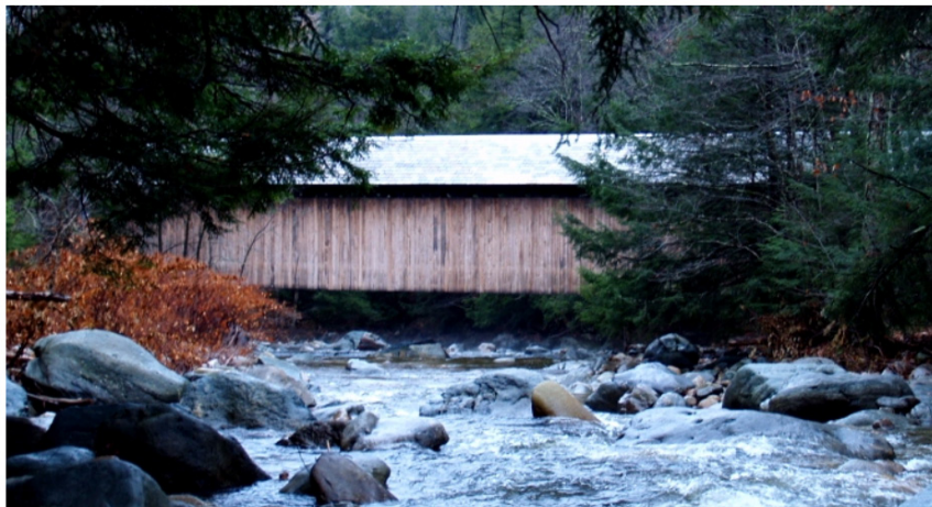
A view of the bridge from the middle of Cold River.
